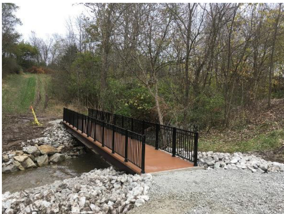
Composite Advantage has developed a new line of standard size fiber reinforced polymer (FRP) trail bridges.
