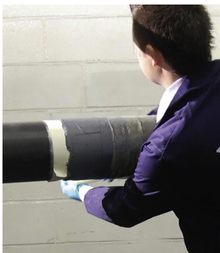
Ten years ago the magazine discussed the use of composites technology in the repair of steel pipes.
